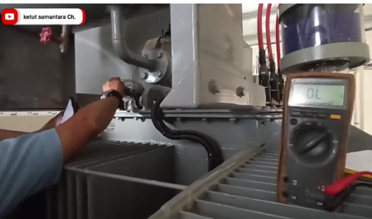
Gambar 6 . Seting komponen pengaman OTI (Over Temperature Indicator)
